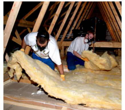
Laying first layer of loft insulation between joists
